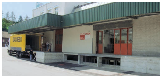
Production facility of ElpoChem
